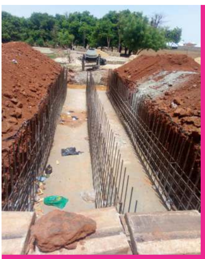
Work on progress before the completion
