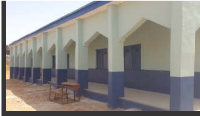
Rehabilitated school in the constituency
