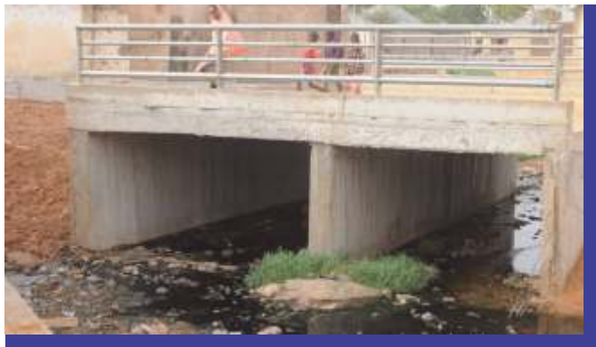
Culvert along eastern bypass, sokoto
