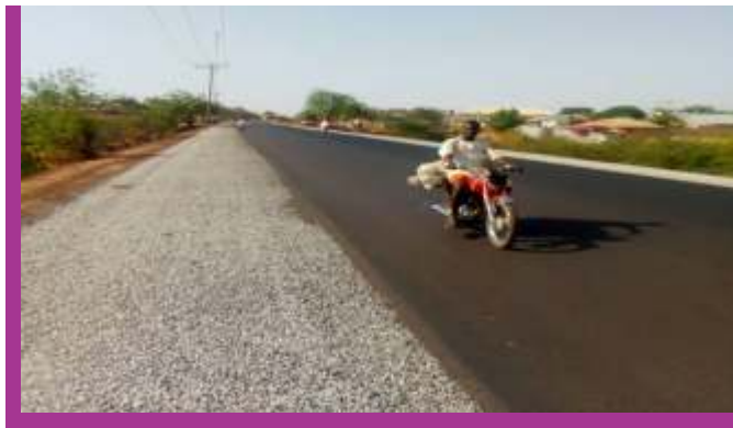
Road rehabilitation along eastern bypass in Sokoto South LGA
