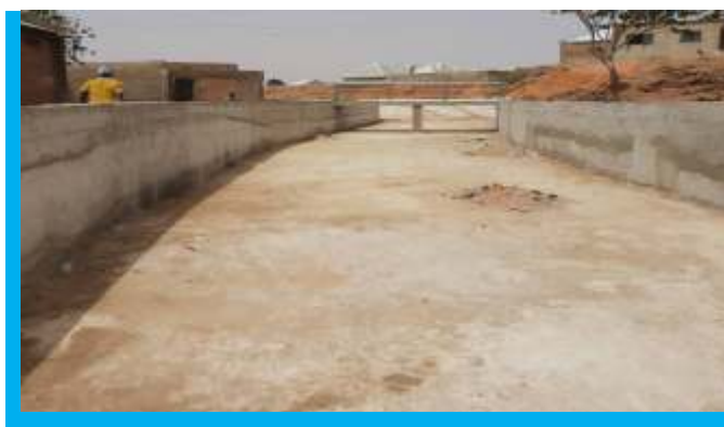
Drainage system along eastern bye pass Sokoto South LGA
