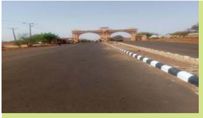
Re constructed Usman Danfodio University Road, Sokoto
